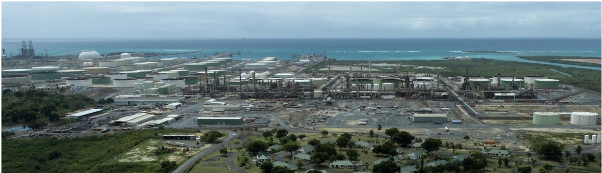
Figure 3. Significant development on St. Croix, such as the Lime Tree Oil Refinery pictured, has impacted water quality and altered natural drainage patterns on the island.
