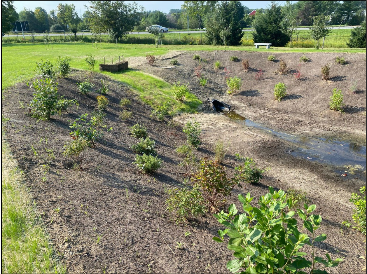
Figure 72. Example photo of a bioretention basin within a gut floodplain.
