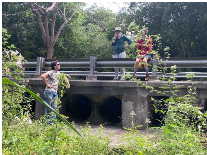
Figure 49. Culverts in the Salt River Bay watershed.
