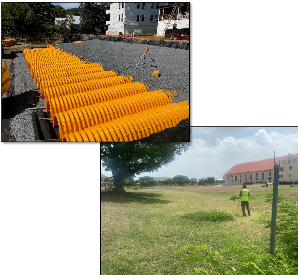
Figure 77. Example photo of subsurface infiltration chambers (above) and major gut channel near the Bethel 7th day Adventist Church (below).
