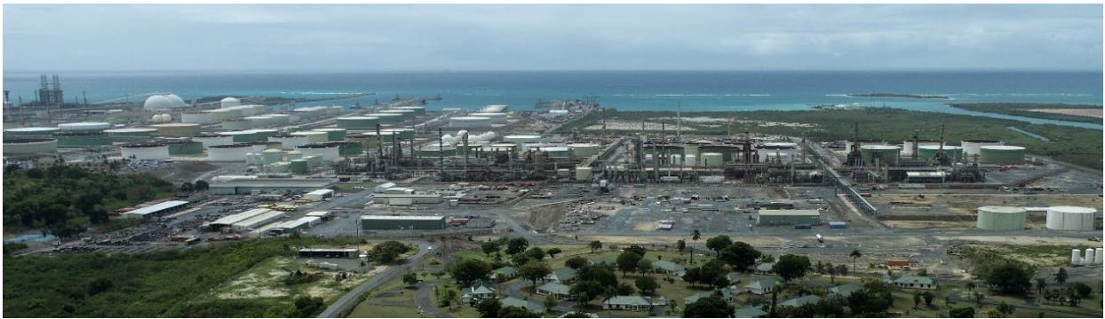
Figure 3. Significant development on St. Croix, such as the Lime Tree Oil Refinery pictured, has impacted water quality and altered natural drainage patterns on the island.
