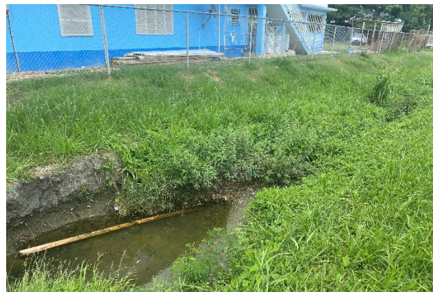
Figure 40. Suspected illicit discharge in gut.
