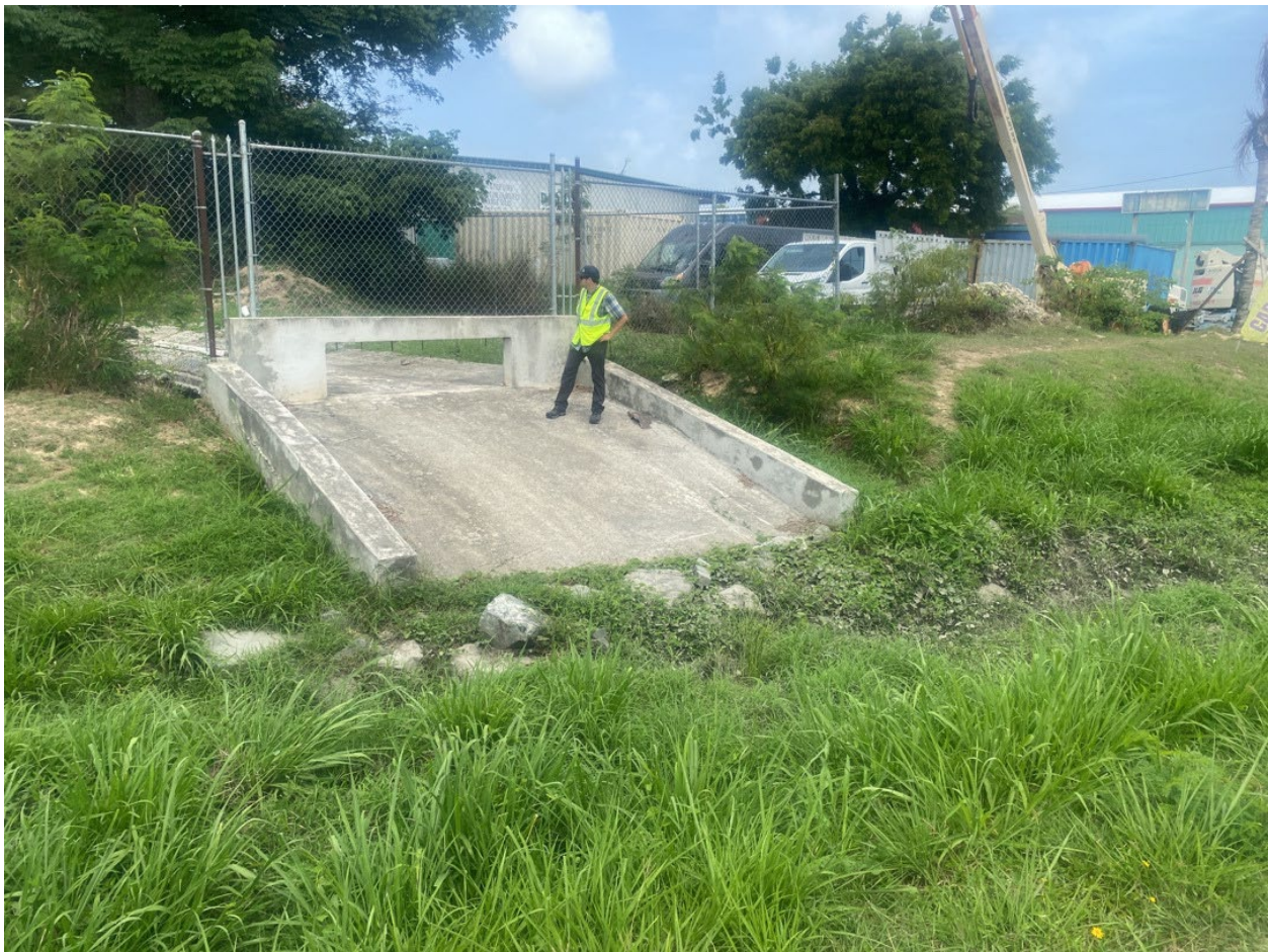
Figure 77. Field assessments were completed across the watershed
