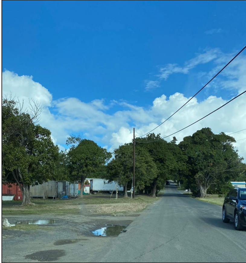
Figure 66. Ponding observed on roads adjacent to the Hov05 monitoring location directly after a storm event.
