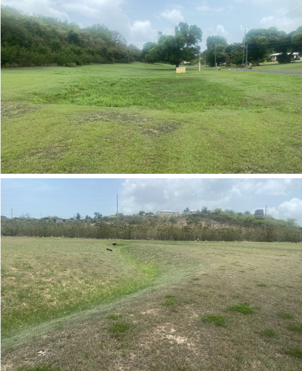
Figure 52. Existing stormwater BMPs in Hovensa. BMP #6 basin (above) and BMP #1 basin (below).
