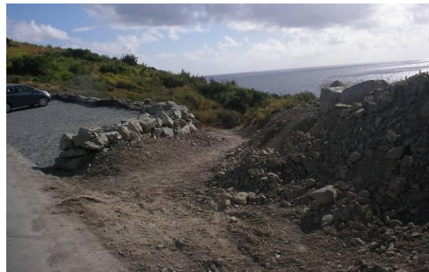
Newly installed parking lot and trailhead.
