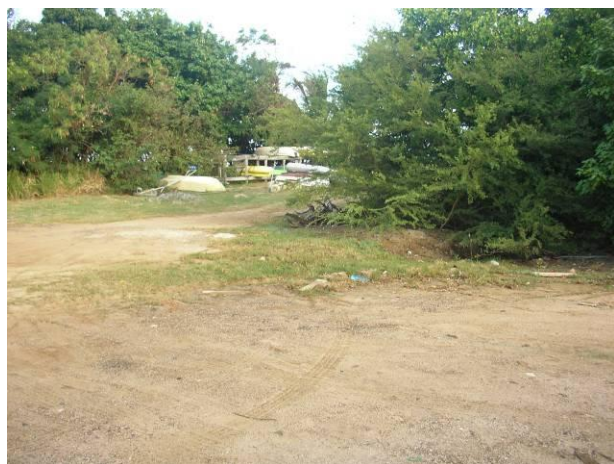
Area for proposed culvert and wetland forebay prior to discharge into gut.
