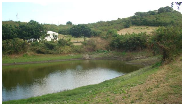
Existing impoundment above headcut.
