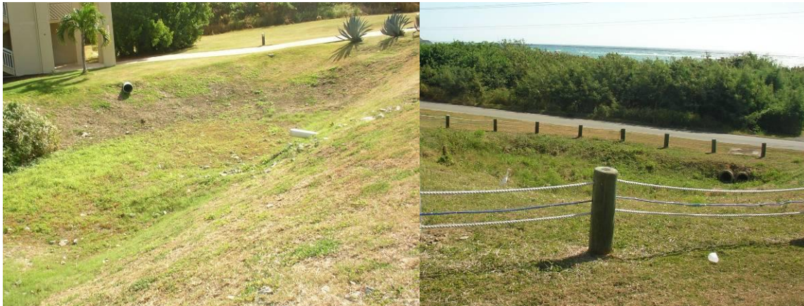
Figure 3. Existing Detention Basins in Turner Hole at Divi
