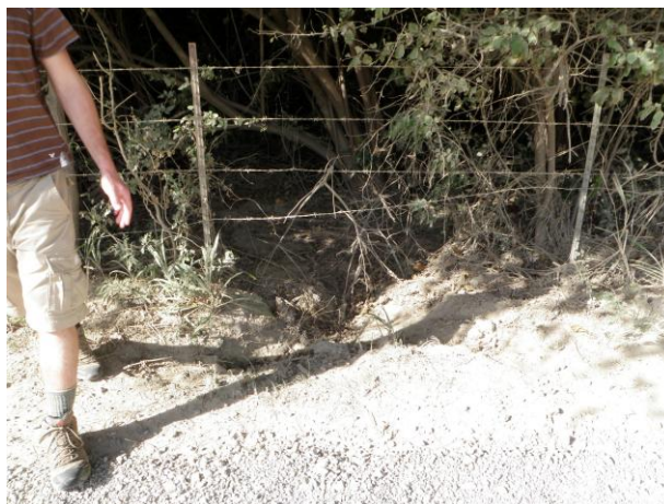
Sediment deposition at outlet location.
