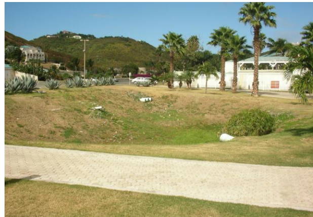
Existing detention basin proposed for modification.
